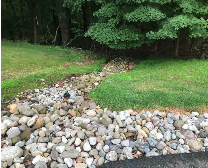
Photo 1 (above): Stone channels extend from the tennis courts and other paved areas into the southern portion of the Preserve, ultimately into Wetland #4.
